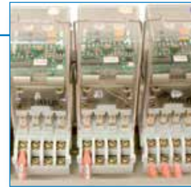
Mors Smitt time delay relays with safety contacts (WNT, weld no transfer) have been selected.
