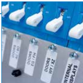
The ultra reliable hydraulic magnetic miniature circuit breakers from Mors Smitt are used.
