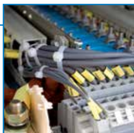
Sturdy wiring and cable layout
