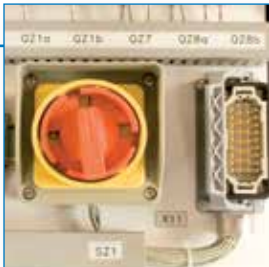
Cable duct, wire numbering printed on the wire and Harting connectors are used.
