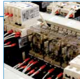
Mors Smitt D-U200 high reliability relays are used.
