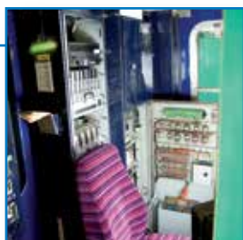
R&D for integration of timing board and relay function into one relay block unit for new and retrofit applications.
