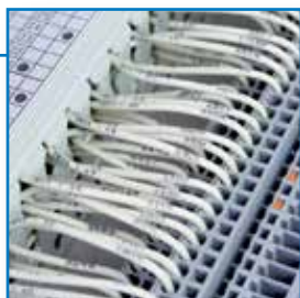
Wire identification by unique, individual printed wires
