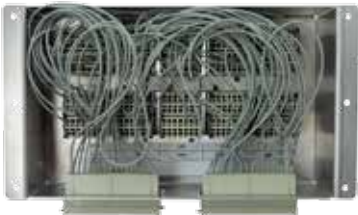
Inside wired relay module
