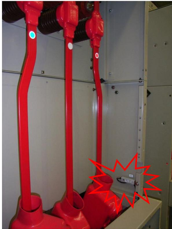
Sensor placement inside the cable termination chamber
