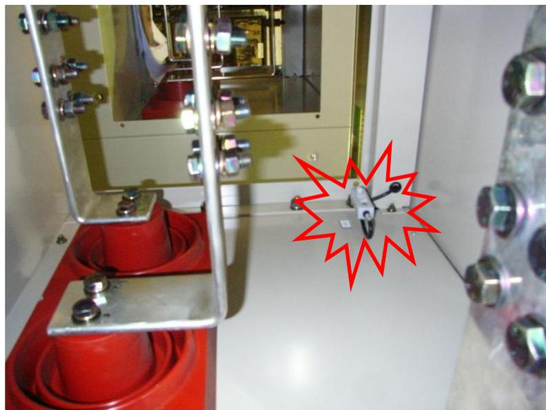
Sensor placement inside the busbar chamber
