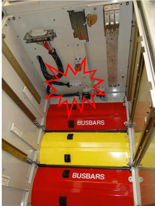
Sensor placement inside the CB racking chamber
