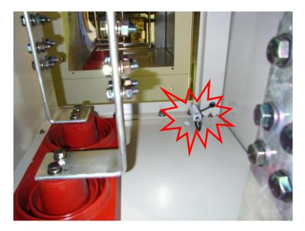
Sensor placement inside busbar chamber
