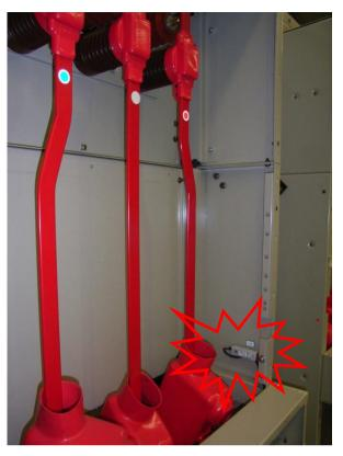
Sensor placement inside cable termination chamber
