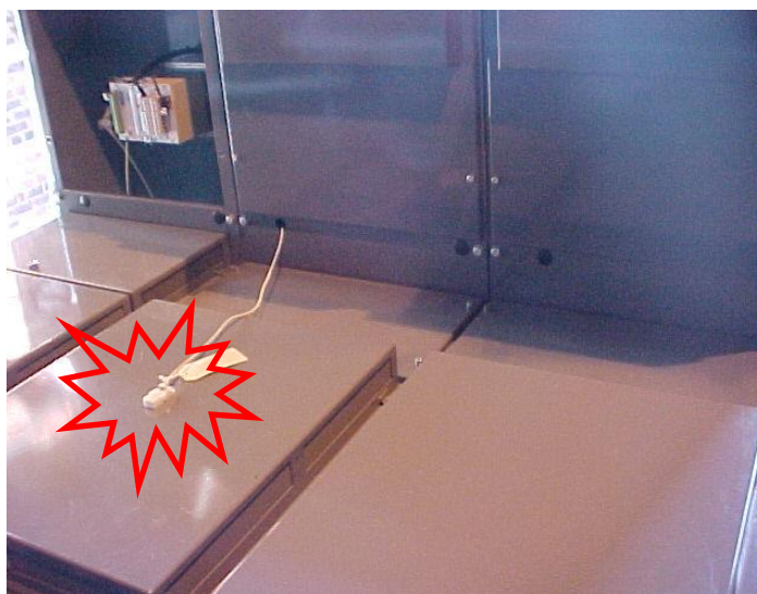
Sensor placement for a Switchgear cable termination chamber (External through Hole Detector)
