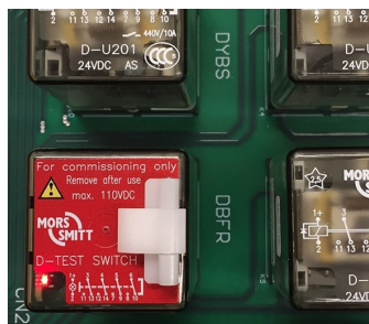
Test for voltage presence: Voltage is present (LED indicator ON)
