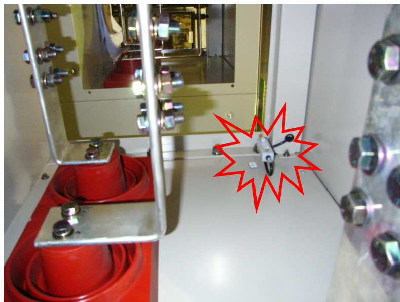
Sensor placement inside busbar chamber
