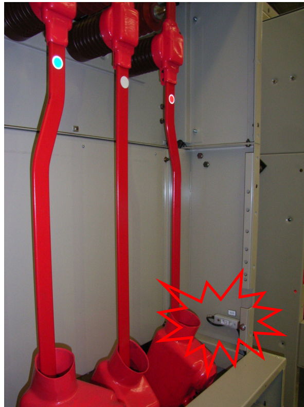
Sensor placement inside cable termination chamber
