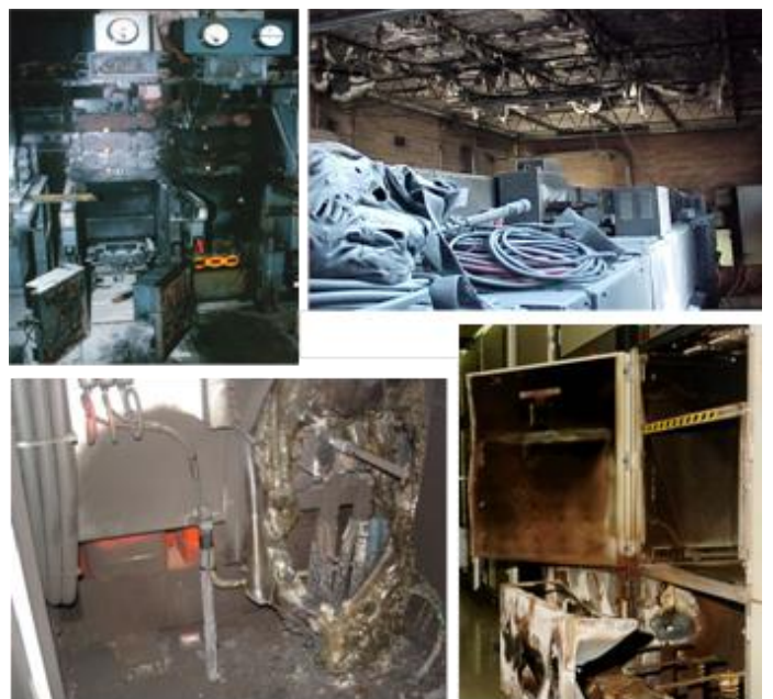
Figure 4: Consequences of arcing faults
