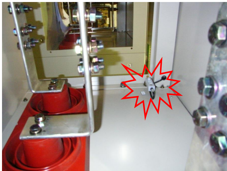
Sensor placement inside busbar chamber
