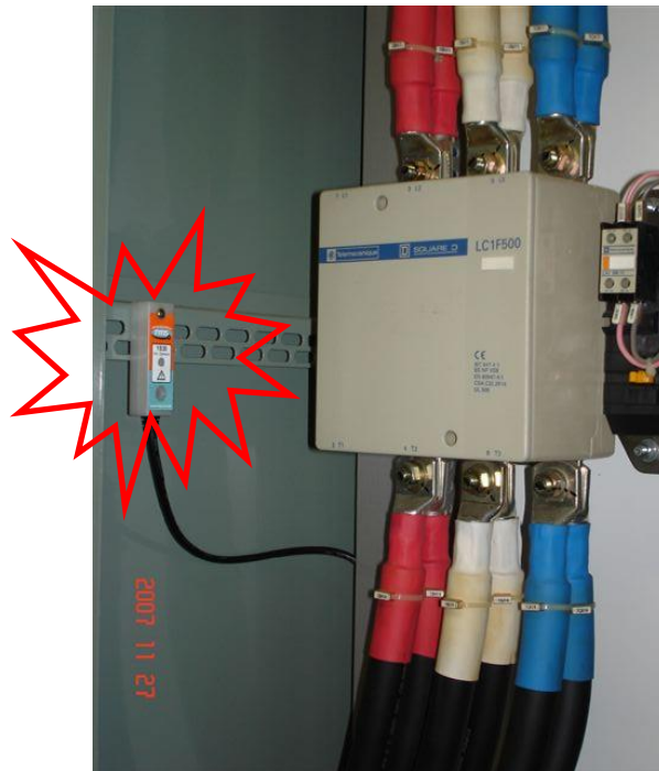
Sensor placement near Low Voltage Contactor for a Variable Speed Drive
