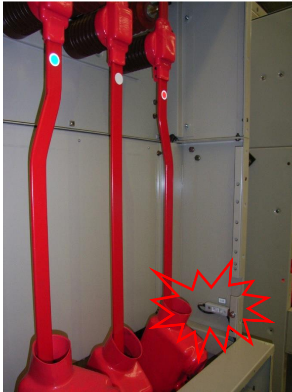
Sensor placement inside cable termination chamber
