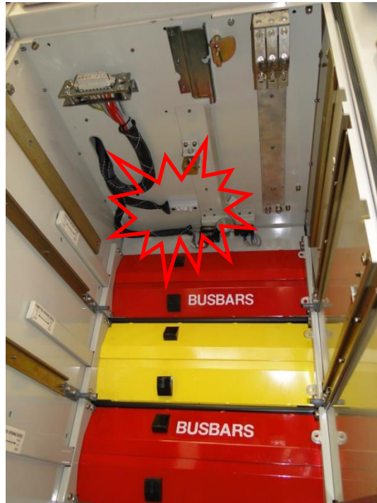
Sensor placement inside CB racking chamber
