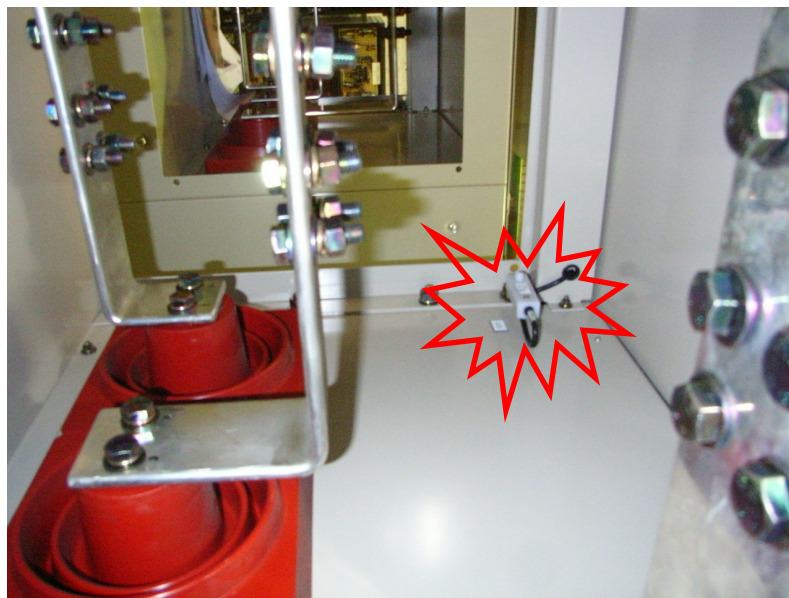
Sensor placement inside busbar chamber
