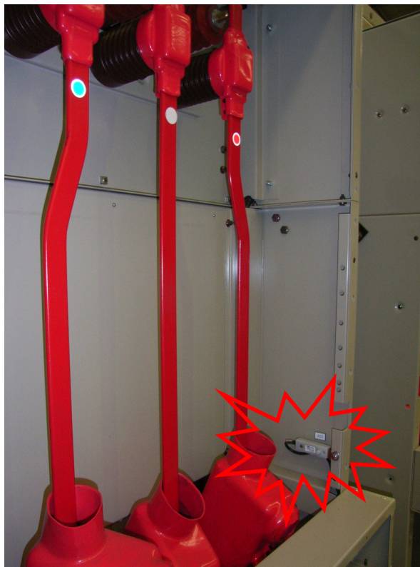
Sensor placement inside cable termination chamber
