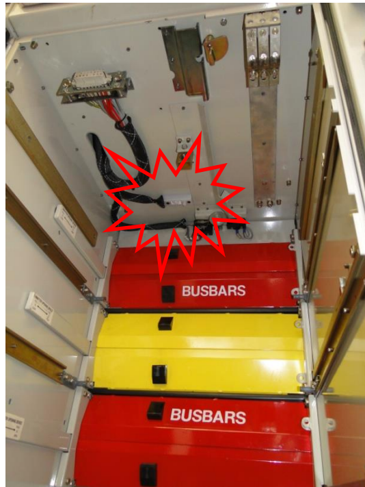
Sensor placement inside CB racking chamber
