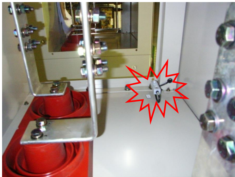
Sensor placement inside busbar chamber
