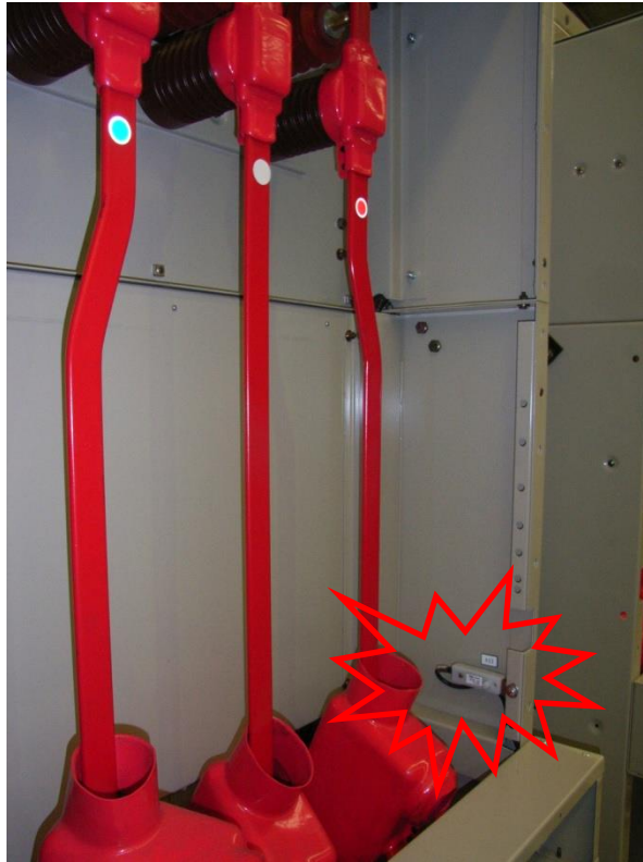
Sensor placement inside cable termination chamber
